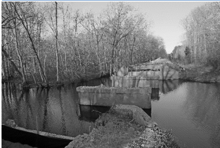
Carson Road (Rte 703) Bridge Replacement
