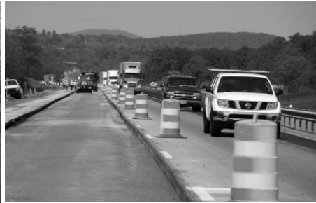
I-81 Pavement Project
