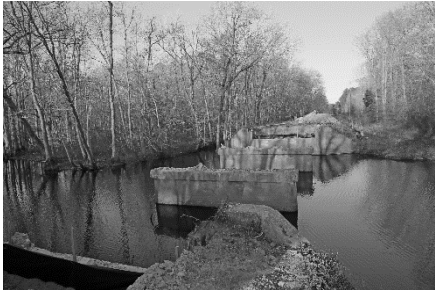
Carson Road (Rte 703) Bridge Replacement
